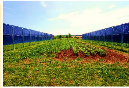
Vertical bifacial solar agrivoltaic system in Europe by Next2Sun.
