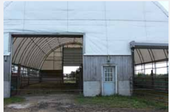
The exterior of Earl Fournier's pack barn. Large overhead doors provide access for equipment as well as ventilation. (Photo courtesy of J. Brown)
