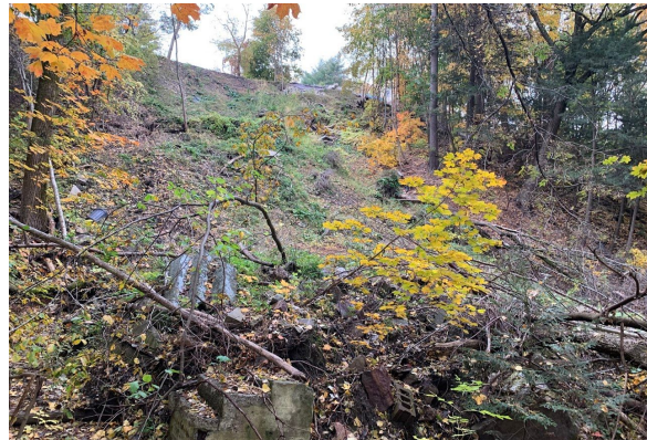
Figure 8: Site of the “Halloween” landslide. Photo taken in Oct 2020
