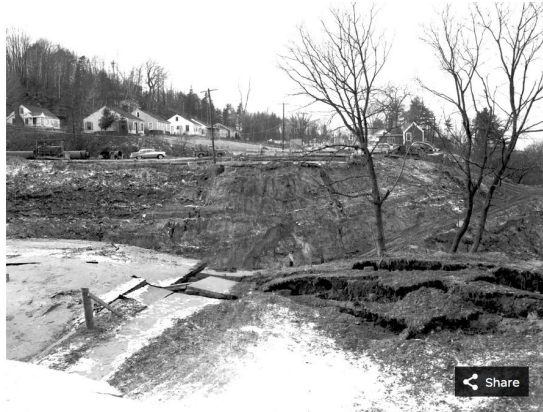
A massive 1955 collapse of the hillside beneath Riverside Avenue in Burlington closed the road and literally undermined decades of work to stabilize the slope. This photograph was taken Dec. 8, 1955 by James Detore to document damage for the American Fidelity insurance company.
