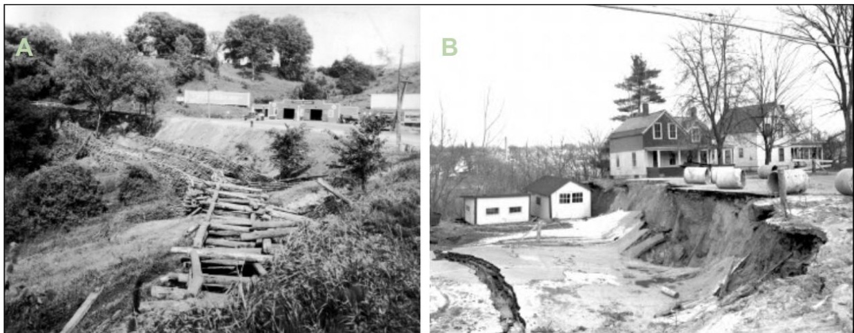
Figure 3: Historic images of Riverside Ave (Source: uvm.edu/landscape ). Image A depicts road widening with wooden shorings and fill in progress between 1930 and 1955. Image B is of the 1955 landslide.
