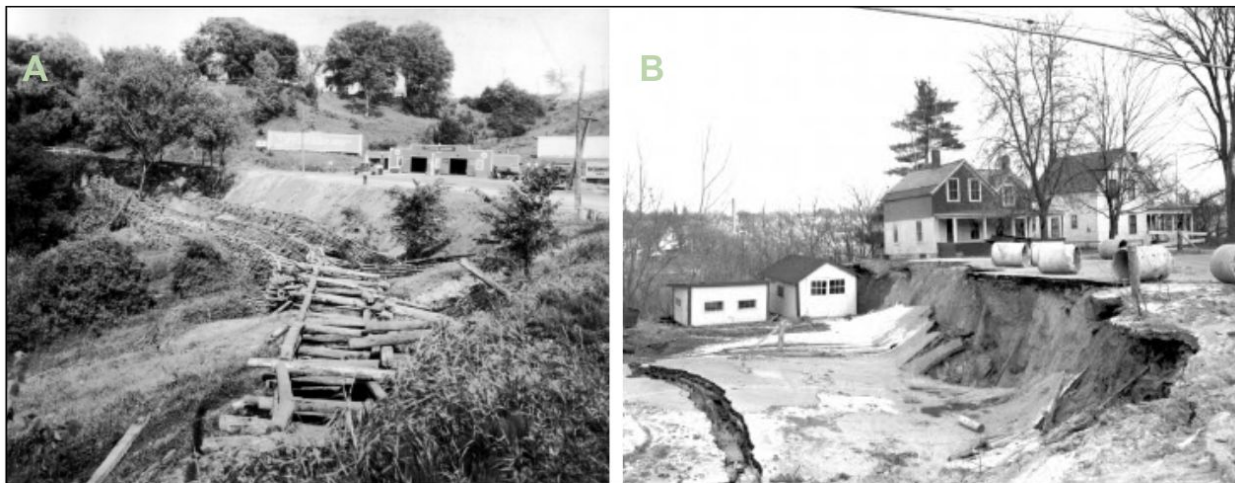
Figure 3: Historic images of Ipswich (Source: uvm.edu/landscape ). Image A depicts road widening with wooden shorings and fill in progress between 1930 and 1955. Image B is of the 1955 landslide.
