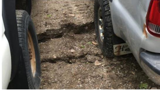
Figure 4: From Burlington Free Press showing a 6-inch gap starting to form, leading to a crack and shortly before the 2019 Halloween night landslide occurs.
