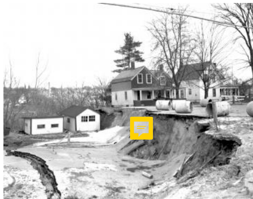
Figure 5: Image taken in 1955 after a landslide on Riverside Avenue significantly lowered a section of the road and small buildings.
