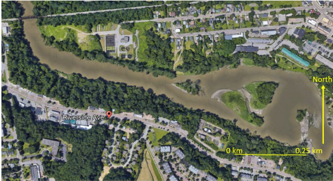
Figure 3: Image of Riverside Avenue taken in 2020.
