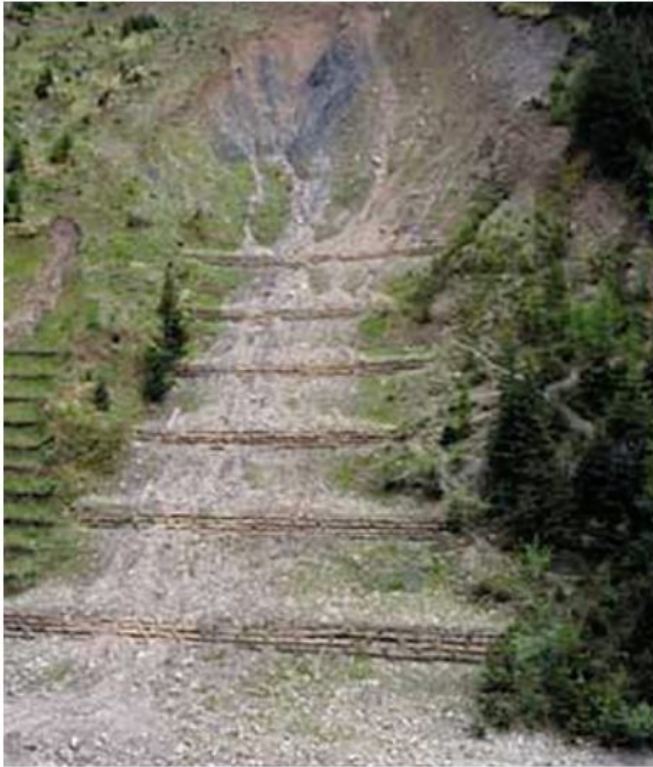
Figure 4: A crib wall check dam (Photo taken in Trafoi, Italy, courtesy of “Erosion Control” Forester Communications, Santa Barbara, CA.) It appears that the sediment storage dams are already filled.
