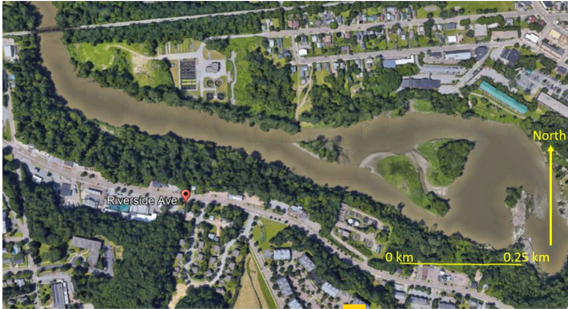
Figure 3: Image of Riverside Avenue taken in 2020.
