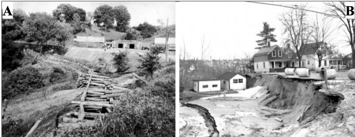
Figure 3: A) Historic photograph of road widening with wooden shorings and fill from early 1930 on the north side of Riverside Avenue. B) December, 1955 Riverside Avenue landslide. Sourced from the UVM Landscape Change Program website. Photo credit: A) L.L. McAllister, B) James Detore
