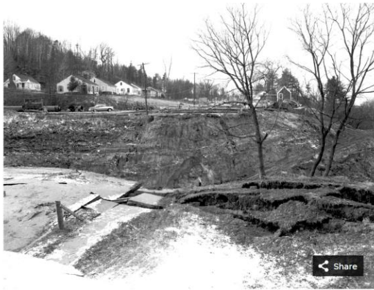
Figure 2: Insurance photo from the historic 1955 landslide that wiped out the middle of Riverside Ave. News reports account the road detour through a landfill. From "History of a Slippery Slope" 2019.
