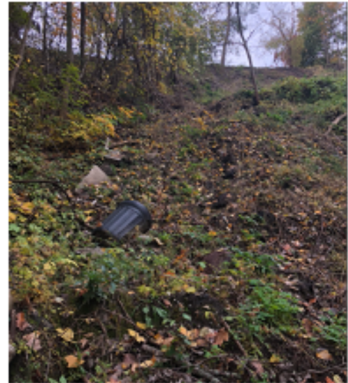
Figure 2: Image of the steep slope where the 2019 landslide occurred. Various debris including trash and concrete are visible (Liviya Kovacevic 2020).
