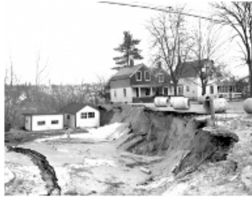
Figure 6: Image taken in 1955 after a landslide on Riverside Avenue significantly lowered a section of the road and small buildings. (UVM Landscape Change Program).
