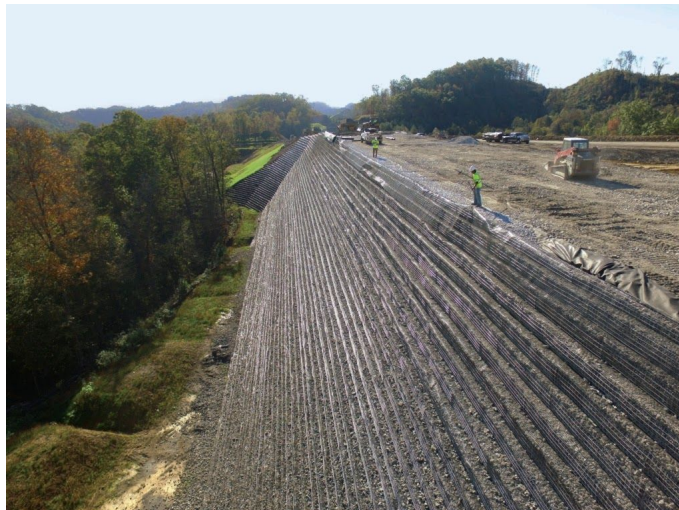
Figure 4: A reinforced soil structure being constructed. Source: (Mandavkar and Weldu, 2019)
