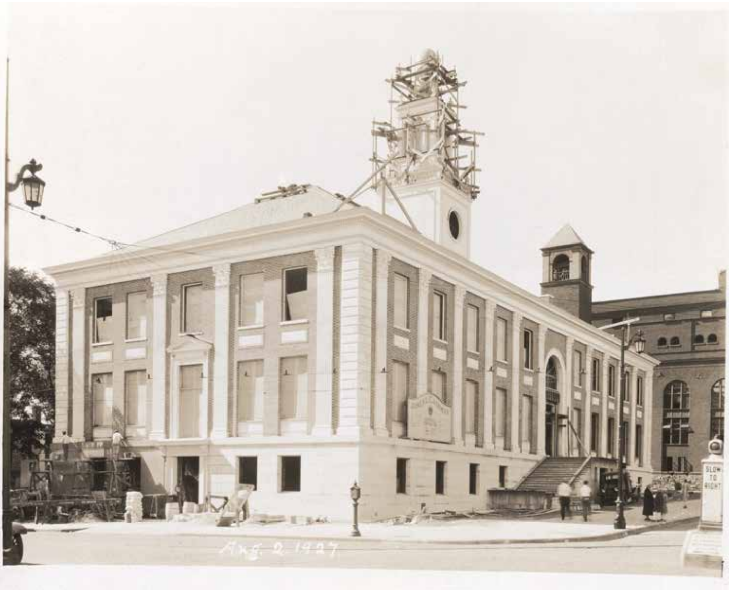
Burlington's colonial revival City Hall under construction in 1927
