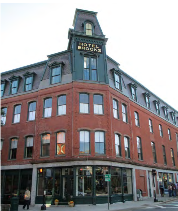
Newly rehabilitated Brooks House stands prominently on Main and High Street in Brattleboro, VT.
