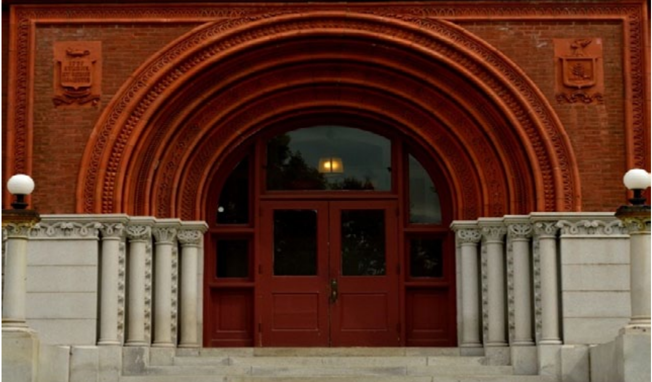
Resting upon a granite base with engaged colonnettes, the Syrian archway surrounding the front entrance of Williams Hall at the University of Vermont is clad in unglazed terracotta tiles.
