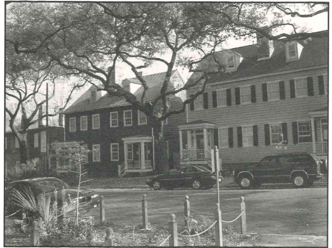
Houses under renovation on Jones Street in Savannah, Georgia (Barb Shubinski)
