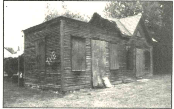
Threatened equipment shed at Elmwood Cemetery, Burlington. (Anne Jennings)
