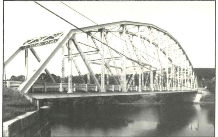
A maintenance poster for Vermont's historic bridges will help bridges such as the Piermont/Bradford Bridge, Bradford, VT, survive. (Bill Thrane)
