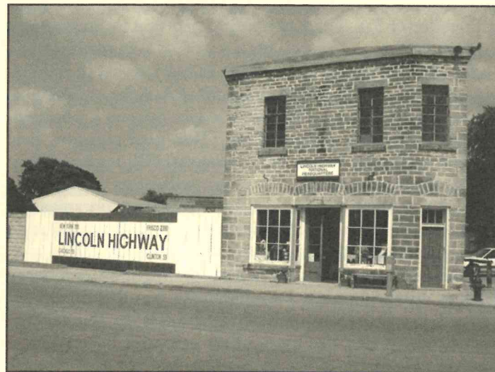
Headquarters of the Lincoln Highway Association, this former dry goods store was built in 1860 by H. I. Lincoln in Franklin Grove, IL.
