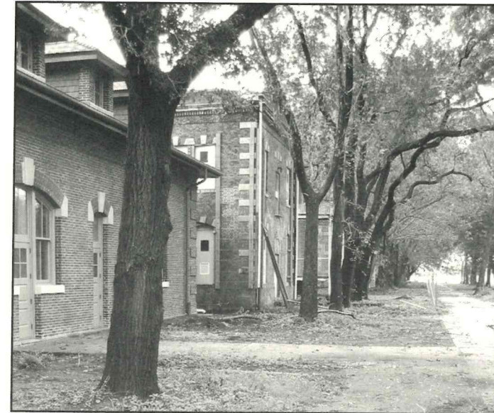
Exterior of hospital buildings. Overgrown vegetation has already been removed as part of the initial stabilization efforts.
