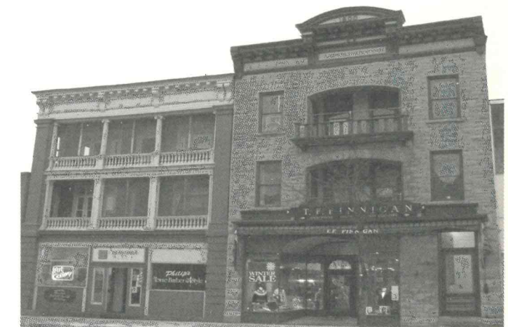
Downtown buildings illustrate the influence of porches on the second and third stories in Saranac.
