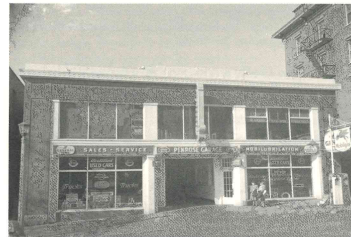
Penrose Garage, 1947, Burlington, Vermont (photograph courtesy UVM Library Special Collections)
