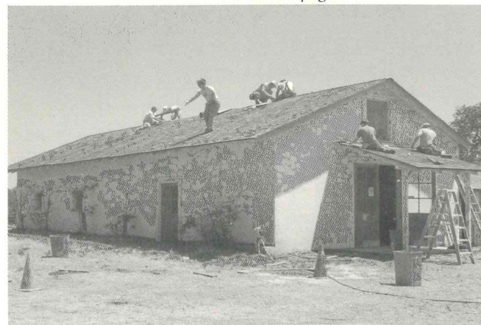
At right: Workers replace asphalt shingles on the carriage barn with cedar shingles.
