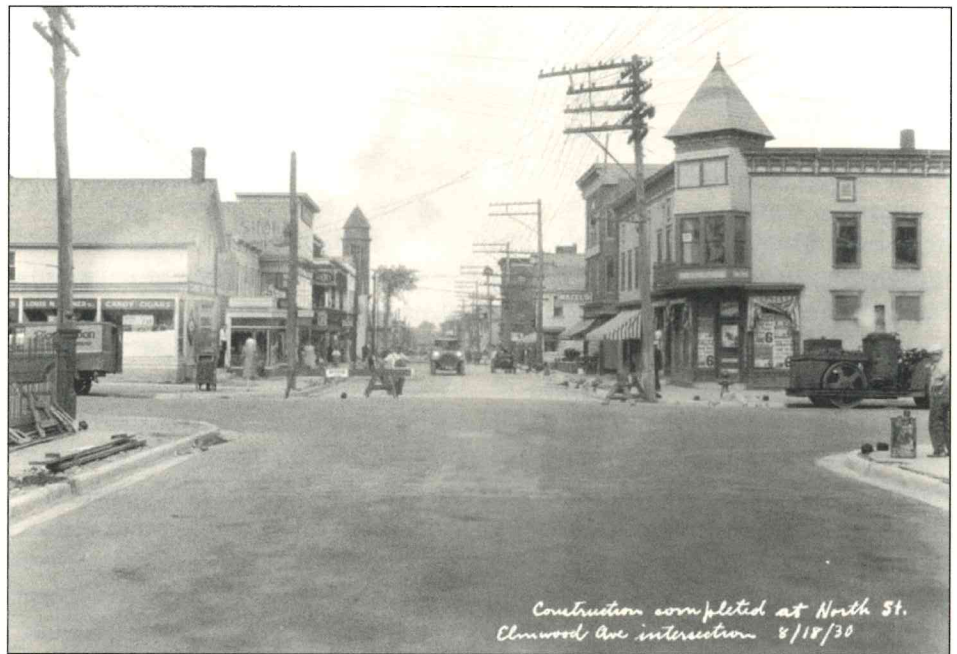
Construction completed at North St. Elmwood Ave intersection 8/18/30 A typical McAllister photograph, looking west down Burlington's North Street. Photo courtesy of McAllister Collection, Special Collections, UVM Libraries.
