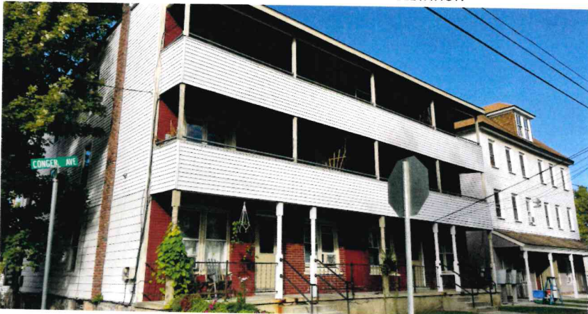
29-33 CONGER AVENUE, LOOKING NORTH-WEST AT PRINCIPAL ELEVATION
