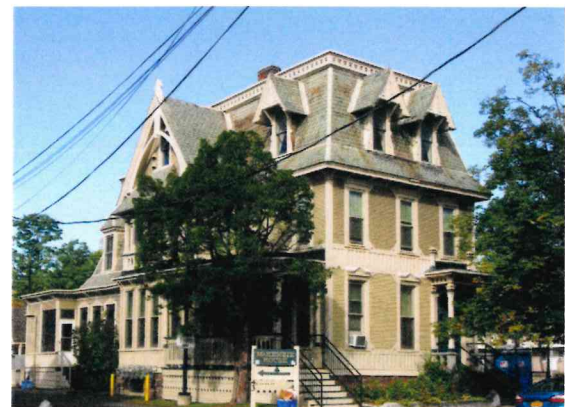
MARTIN L. KELSEY HOUSE, 43 ELMWOOD AVENUE
