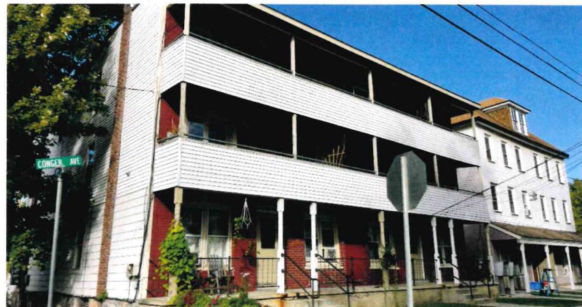
29-33 CONGER AVENUE, LOOKING NORTH-WEST AT PRINCIPAL ELEVATION
