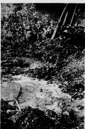
Workers apparently deposited debris from a landfill on the Winooski River. A landslide resulted and the debris slid into the Winooski River.
