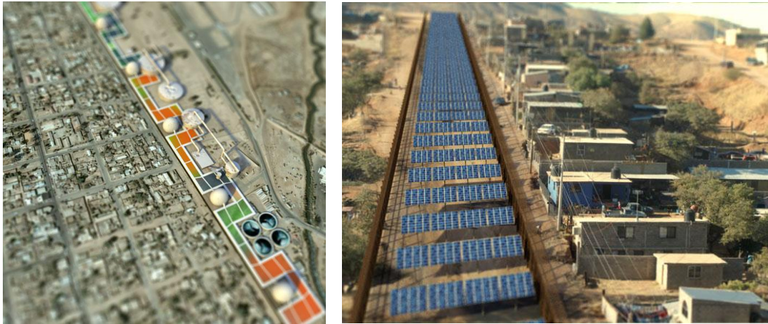
Right. A 20 million-gallons/day wastewater treatment facility on the border between Mexicali, Mexico and Calexico, California. Left. One square foot of solar energy production along the border can power a dishwasher for a year. Border Wall as Architecture.
