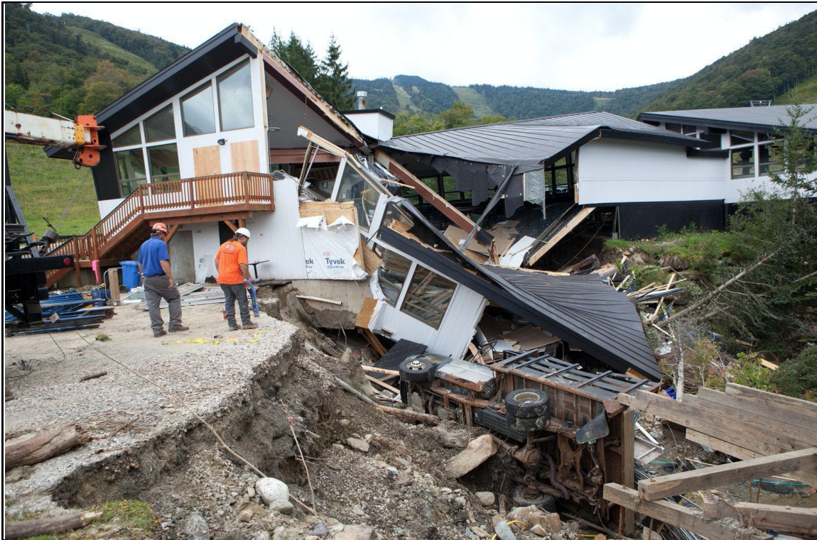
Figure 8-14: Devastated infrastructure due to Tropical Storm Irene in Killington, VT (Inside Climate News, 2016)
